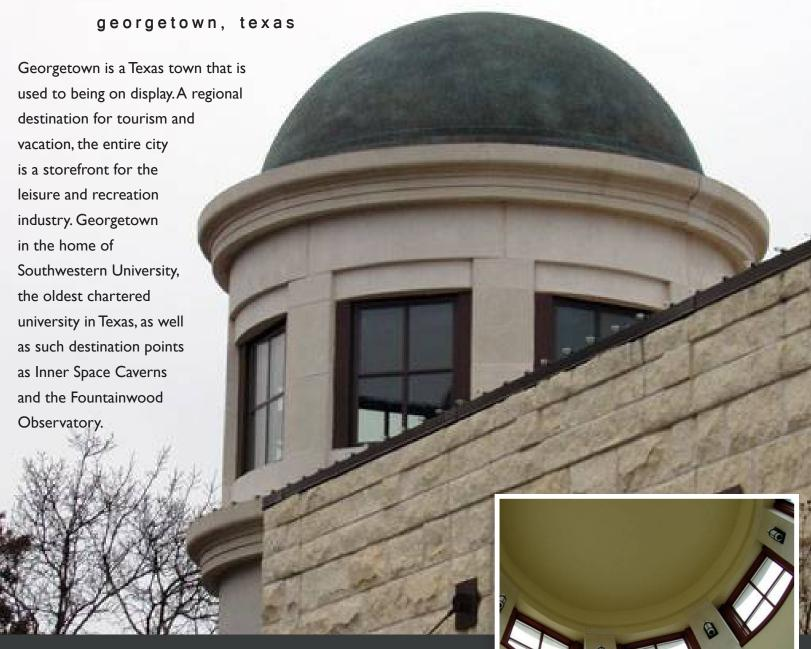
Stromberg was called in to provide cornice and paneling for the Council Chambers when they were built in 2003. The Stromberg elements were composed of wet cast concrete and formed to exacting standards to fit the unusual turret feature of the building. Stromberg Architectural Products has over 30 years of
